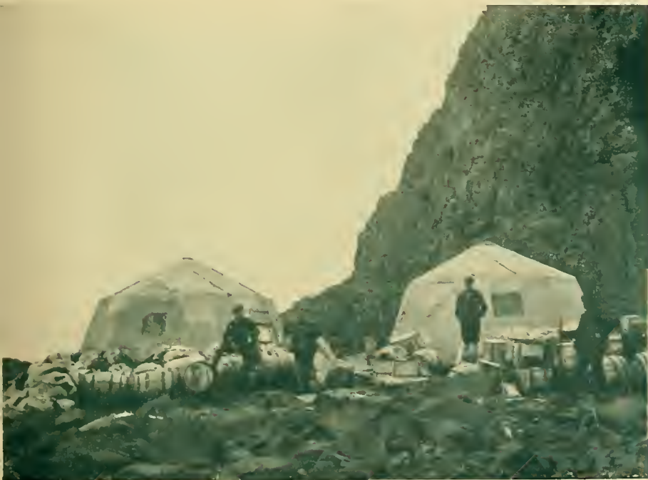
THE TWO HOUSES ON BASS ROCK
